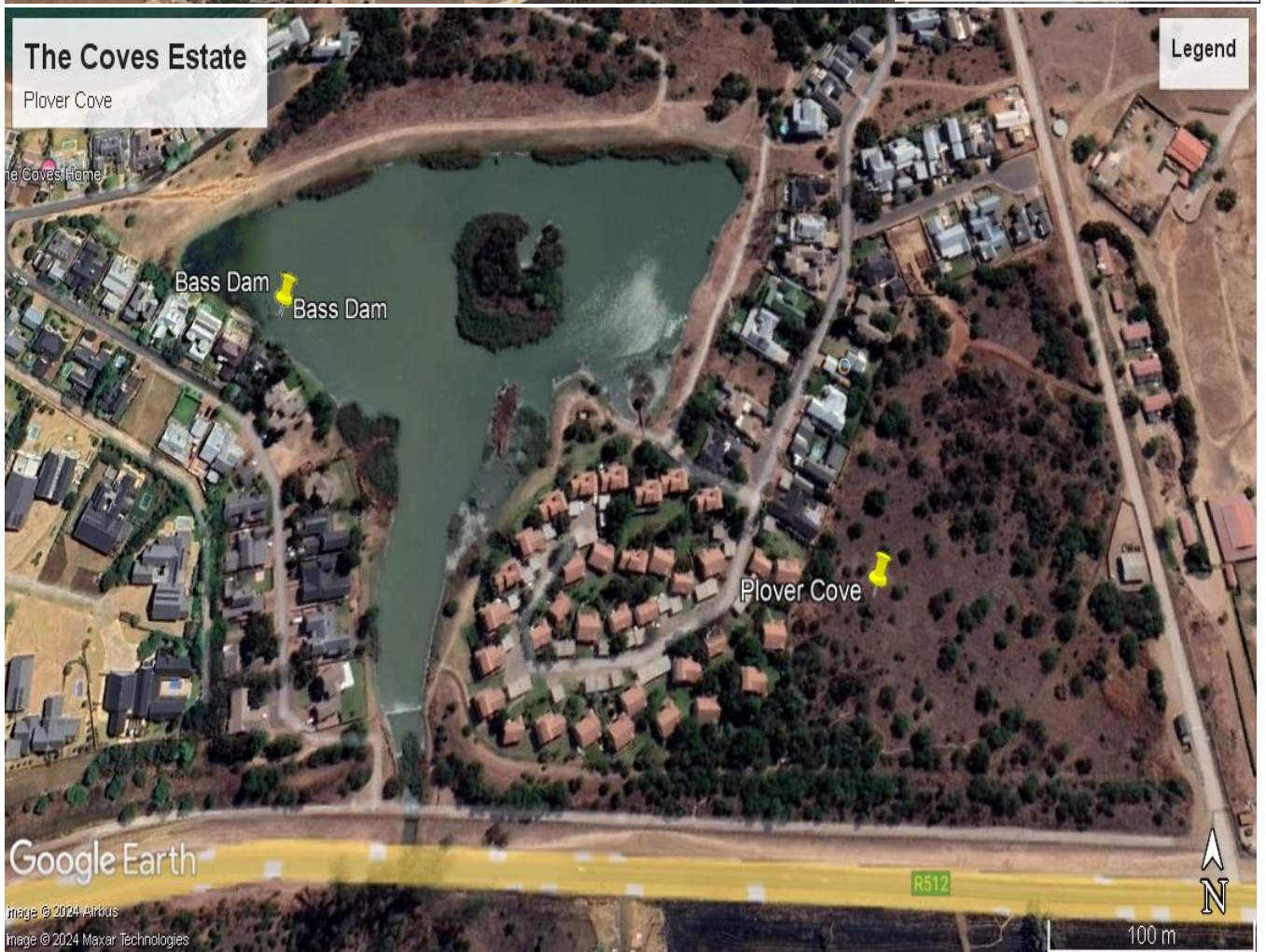
Aerial view of Plover Cove & Bass Dam
